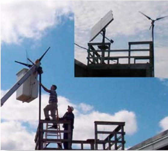
Installing the Wind Generator and Solar Array
